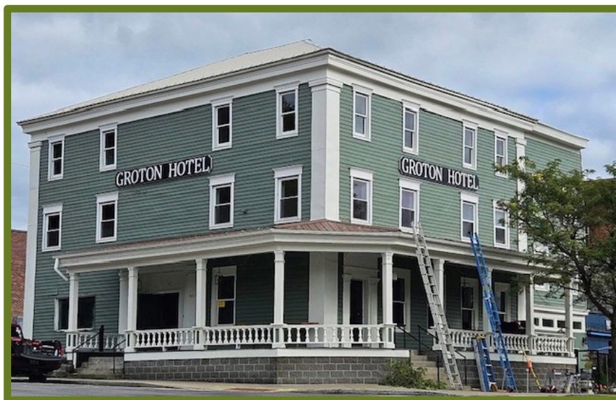
Image: Groton Hotel, Main Street 2026. Source: Thoma Development Consultants
