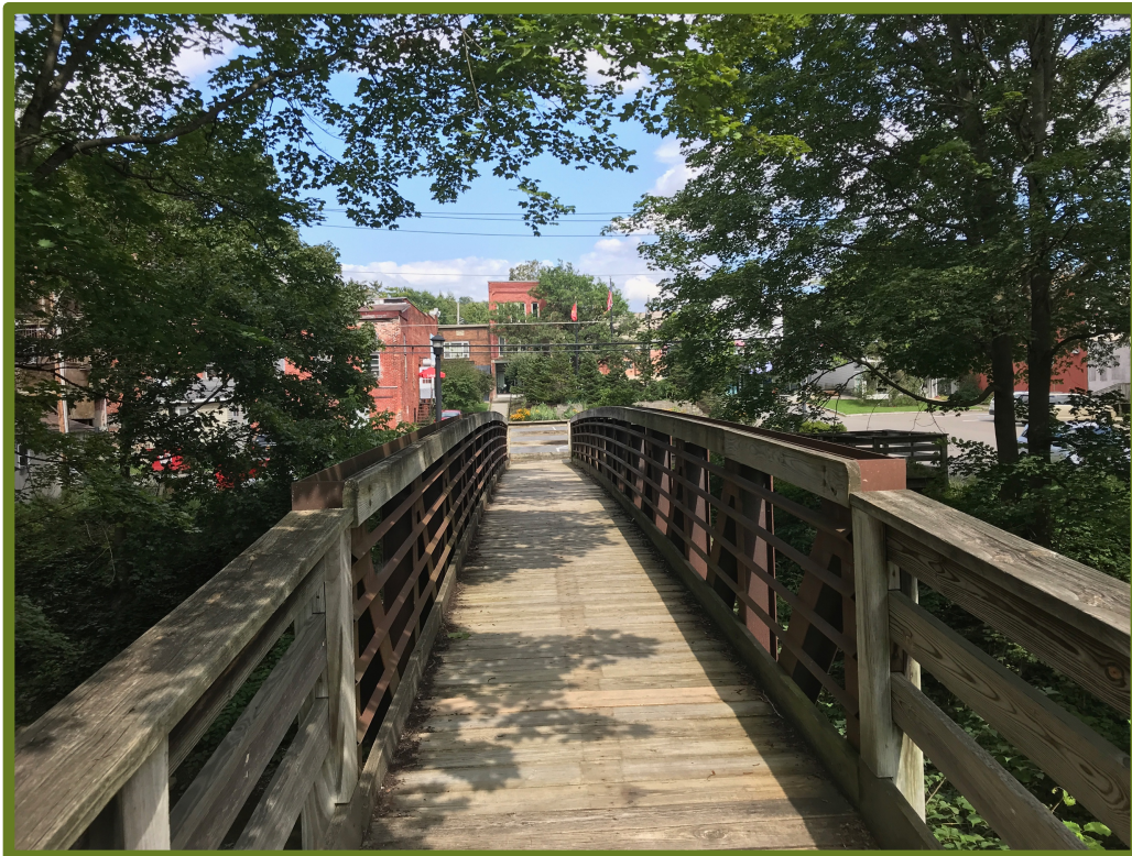
Image: Pedestrian Bridge over the Owasco Inlet in Downtown. Source: Village of Groton
